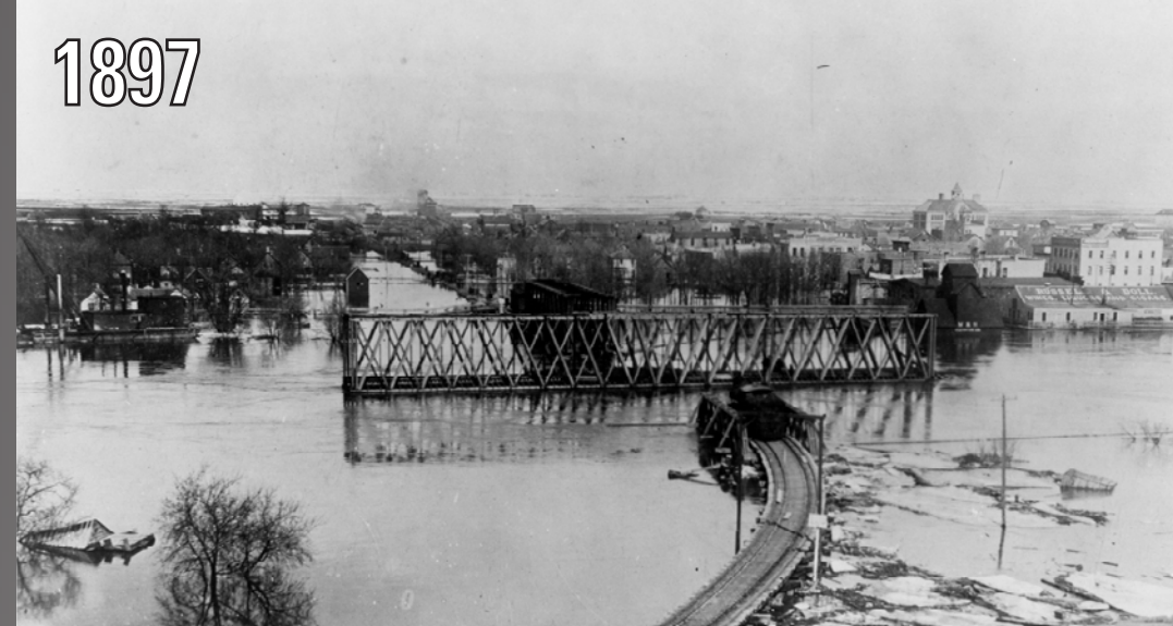
View of East Grand Forks, Minn., during Red River flood of 1897. Center span of Northern Pacific Railroad bridge pivoted horizontally to allow ice to flow past. Engines are parked on stationary spans to weigh down bridge
