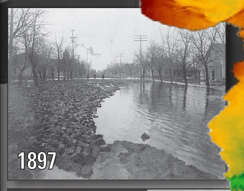
▲ Wooden blocks that once paved the streets of Fargo, N. Dak., piled up during Red River flood of 1897 (Photo from Institute for Regional Studies, North Dakota State University, Fargo 2006.83.19) Red Owl Super Market in flooded area of Fargo, N. Dak., during Red River flood of 1943 (Photo from State Historical Society of North Dakota 0378-015)
