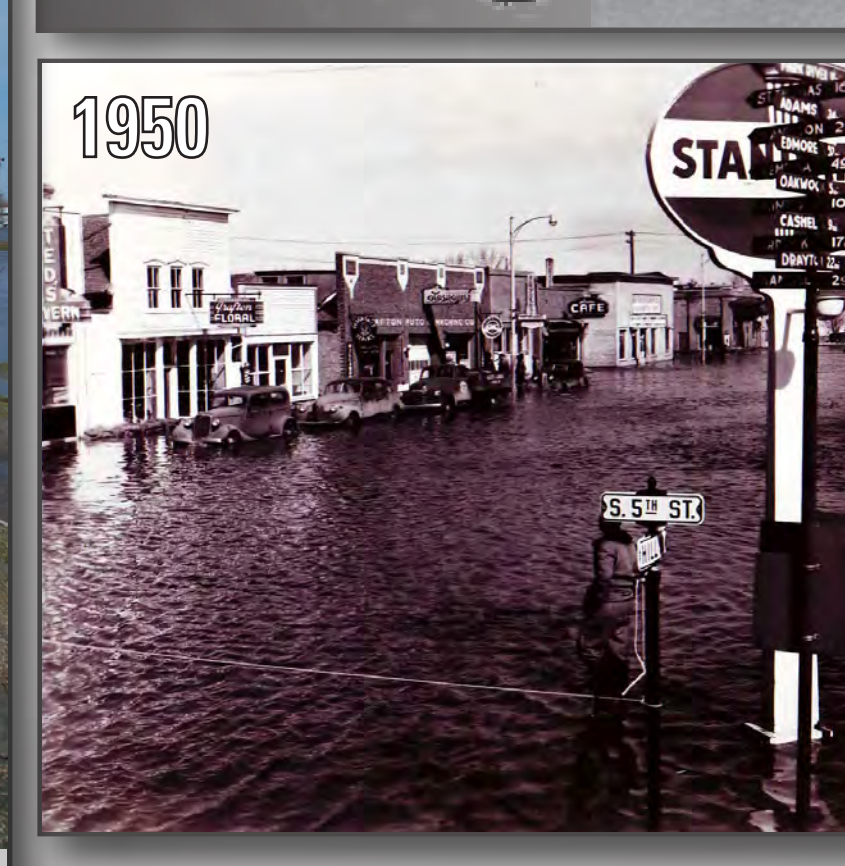
Corner of Fifth Street and Hill Avenue in Grafton, N. Dak., during Park River flood of 1950
