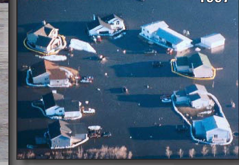
Diked homes at Grand Forks, N. Dak., during Red River flood, spring 1997
