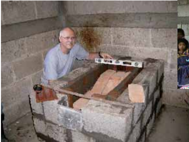
A volunteer is building a stove that will be ventilated to reduce the smoke inside a house.
