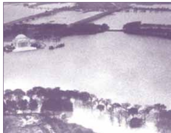
1942 flood damage on the National Mall
