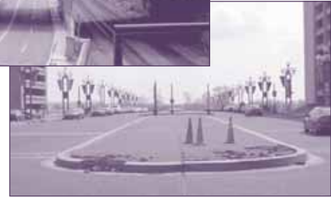
Existing conditions at Banneker Overlook along 10th Street, NW
