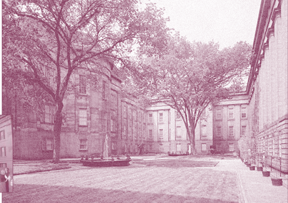
1968 Historic American Buildings Survey (HABS) photograph shows historic courtyard landscape prior to its demolition.
