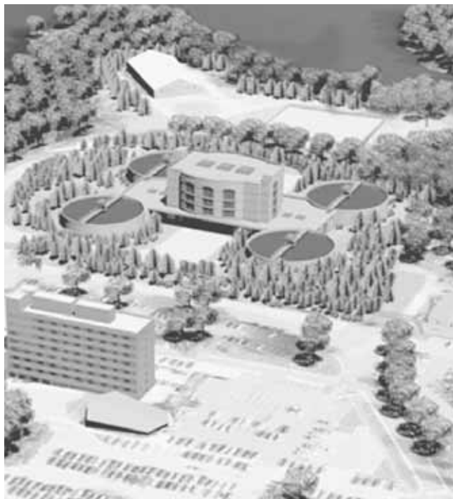
The Commission approved a new water treatment facility and related improvements at the Dalecarlia Water Treatment Plant operated by the Washington Aqueduct.
