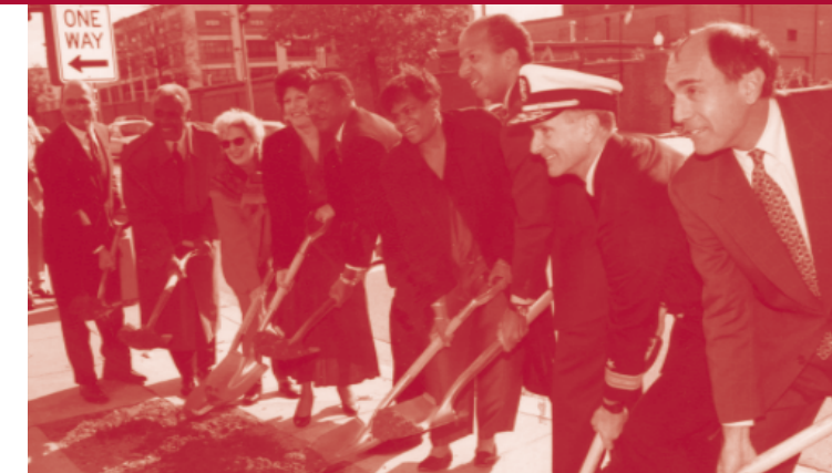
CHAIRMAN GANTT, MAYOR WILLIAMS, AND OTHER FEDERAL AND CITY OFFICIALS BREAK GROUND FOR STREET IMPROVEMENTS ON M STREET, SE.
