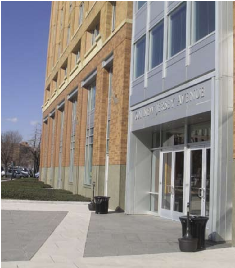
Federal Trade Commission Satellite Building 601 New Jersey Avenue, N.W., Washington D.C.
