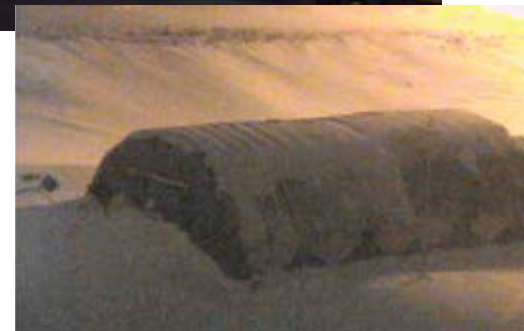
center: Habitat Data Center
