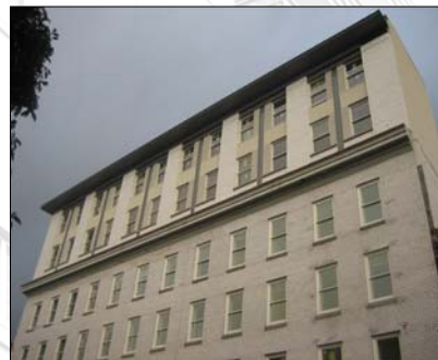
The Estate – renovation completed in December 2007
