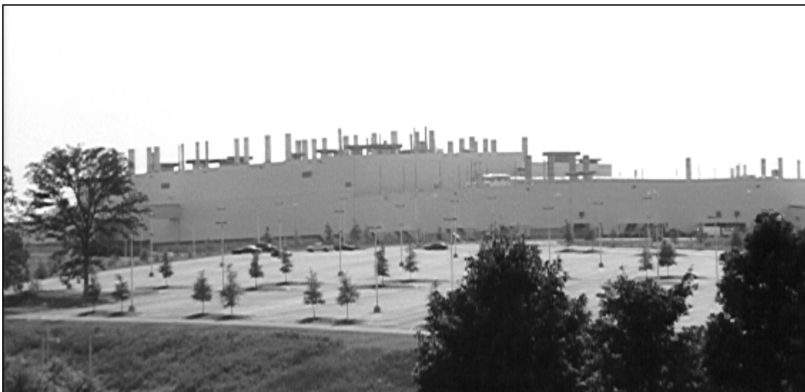
The BMW assembly plant
