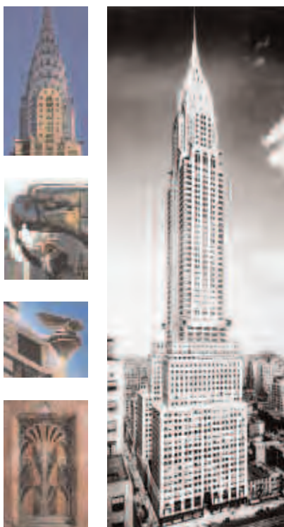
William Van Alen (1883–1954), The Chrysler Building , 42nd Street and Lexington Avenue, New York, 1926–1930. Steel frame, brick, concrete, masonry, and metal cladding, height 1046 ft. (318.82 m.).
