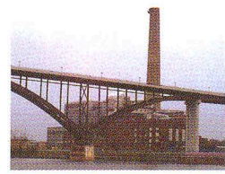
* Xcel High Bridge Plant
