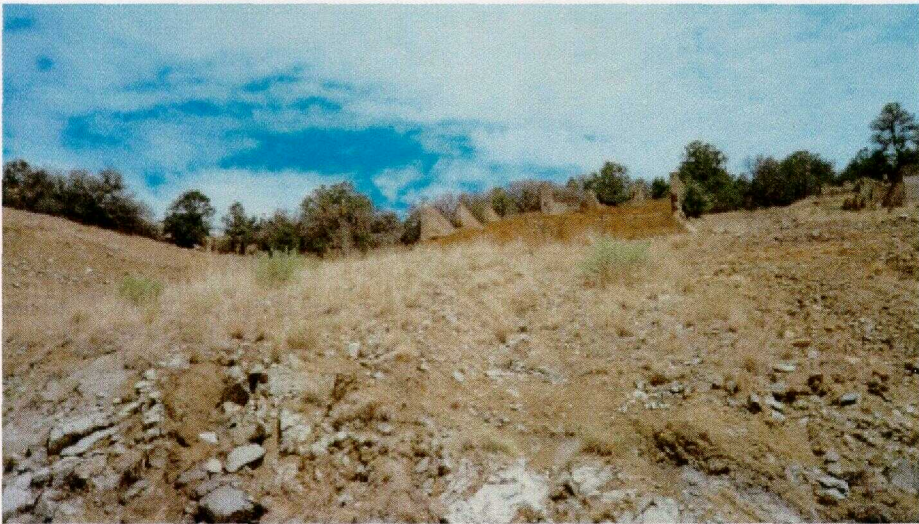
Photo 7: Vegetation at base of Cleveland Mill Building, July 17, 2002
