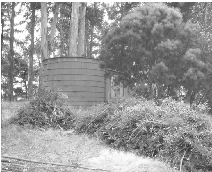
Water tank on East Marin Island USFWS
