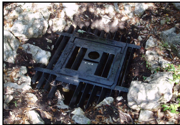
Gated entrance to cave to protect endangered Karst invertebrates, San Antonio, Texas
