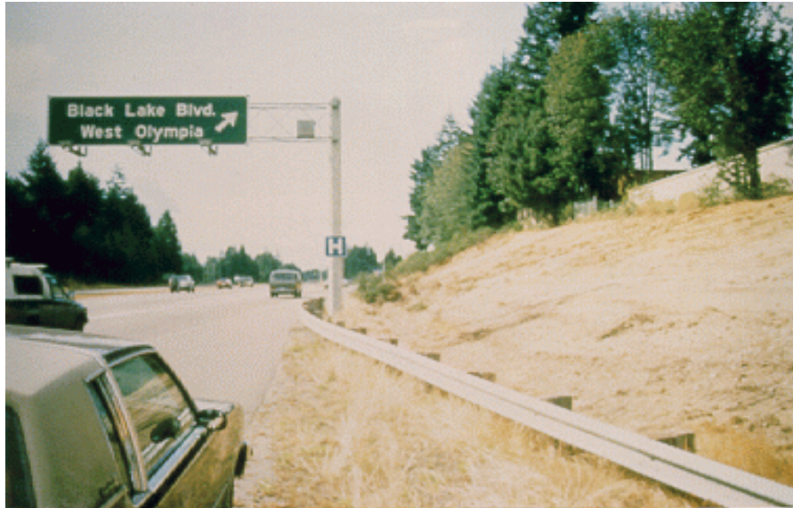
Figure A-1. Black Lake Interchange, WSDOT Olympia, WA - Prior to Construction
