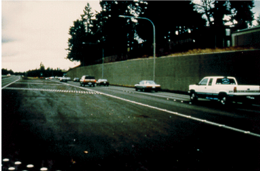
Figure A-3. Black Lake Interchange, WSDOT Olympia, WA - Completed Soil Nail Wall Project
