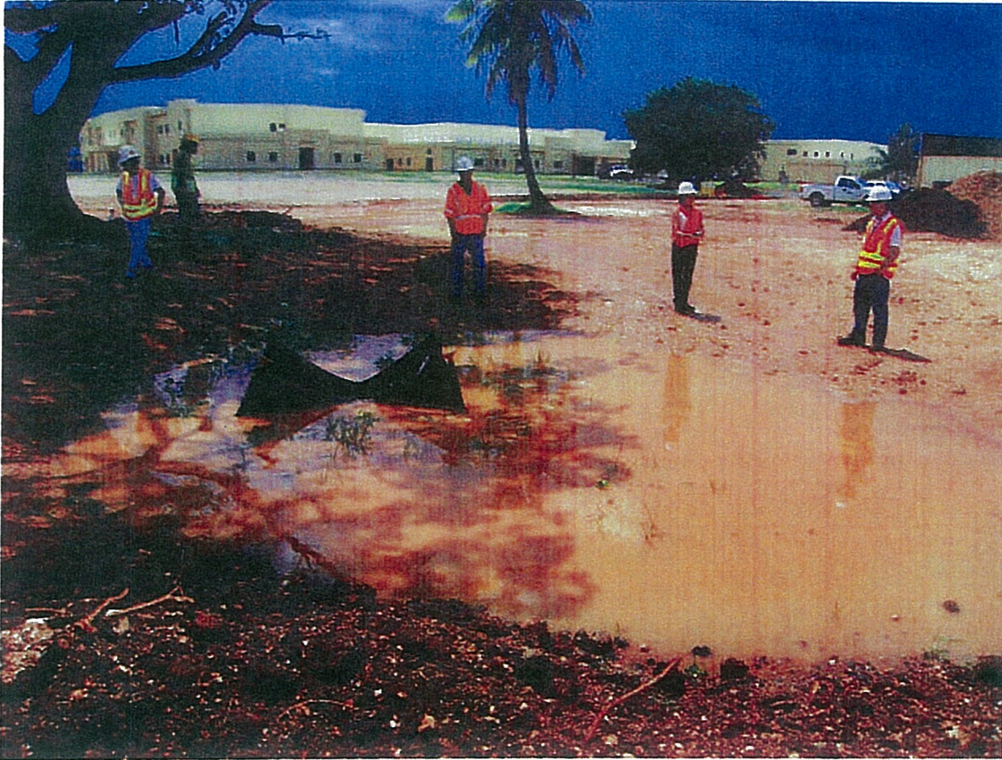
USN Naval Base Guam, CGP Inspection of McCool School Project, 7/16/08 IMG_0014
