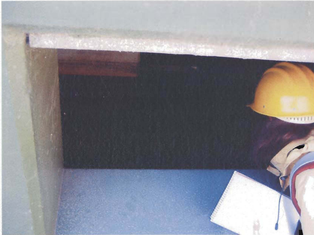
Figure 9: Chlorination chamber beneath FFRs.
