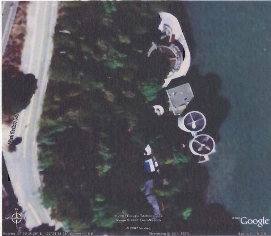
Figure 1: Aerial view showing the location of SMCSD WWTP in Sausalito, California.
