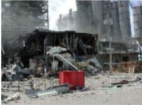
Explosion at a Formosa Plastics Corporation PVC Plant
