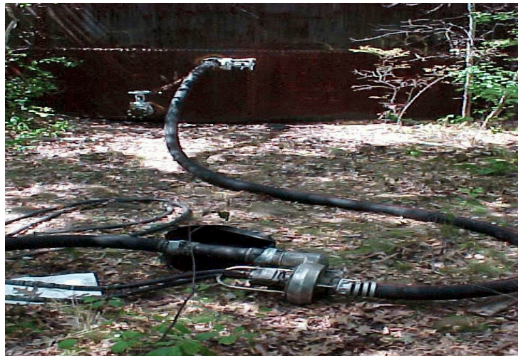
Oil is pumped out of an abandoned tank at the Royal Mills site in Rhode Island.
