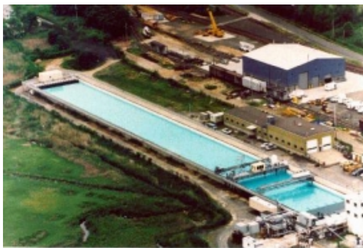
Aerial view of the Ohmsett oil spill test facility in Leonardo, New Jersey—its 2.7 million gallon tank can simulate a variety of response conditions.
