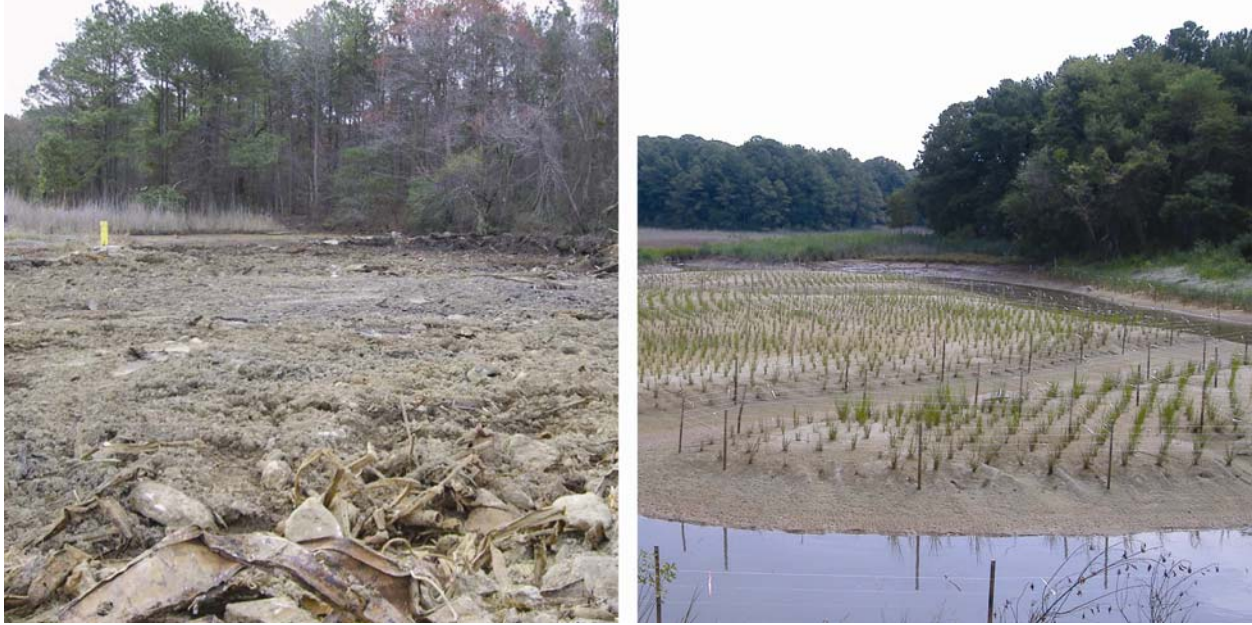
Figure 4-1: Before and after photographs of Naval Amphibious Base Little Creek in Virginia, where the remediation team converted a landfill into a tidal wetland. See Appendix A for additional information. Photographs courtesy of Bruce Pluta, EPA Region 3.
