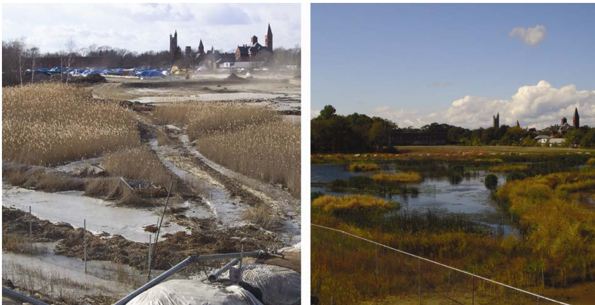
Figure 2-1: Before and after photographs of the Atlas Tack Superfund Site in Massachusetts where the remedy resulted in preservation of wetland sediment and created a functioning wetland. See Appendix A for additional information. Photographs courtesy of Elaine Stanley, EPA Region 1.
