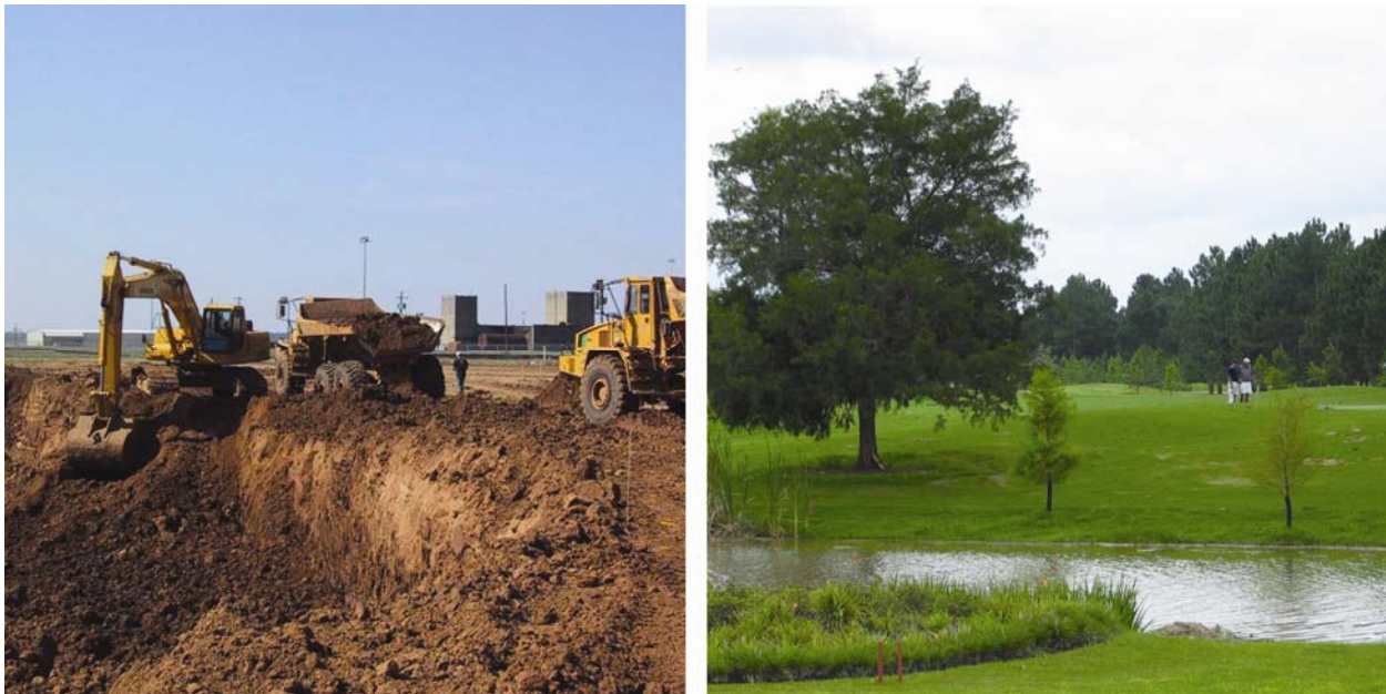
Figure 2-2: Before and after photographs of England Air Force Base in Louisiana where contaminated areas were excavated and became part of the Audubon Trail, providing habitat and a stopping point for migratory birds. See Appendix A for additional information. Photographs courtesy of RCRA Corrective Action Program.
