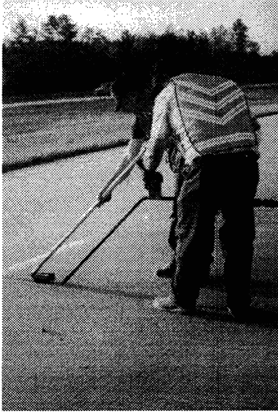
Figure 18. Overbanded sealant installation.
