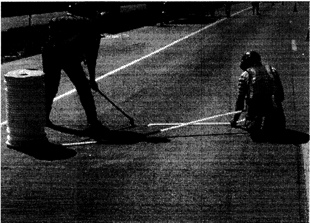
Figure 15. Backer rod installation.
