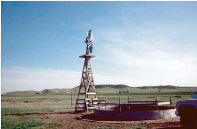
Windmill-powered well and livestock-watering tank, Platte County, Wyoming (Photograph courtesy of J.P. Mason, U.S. Geological Survey.)
