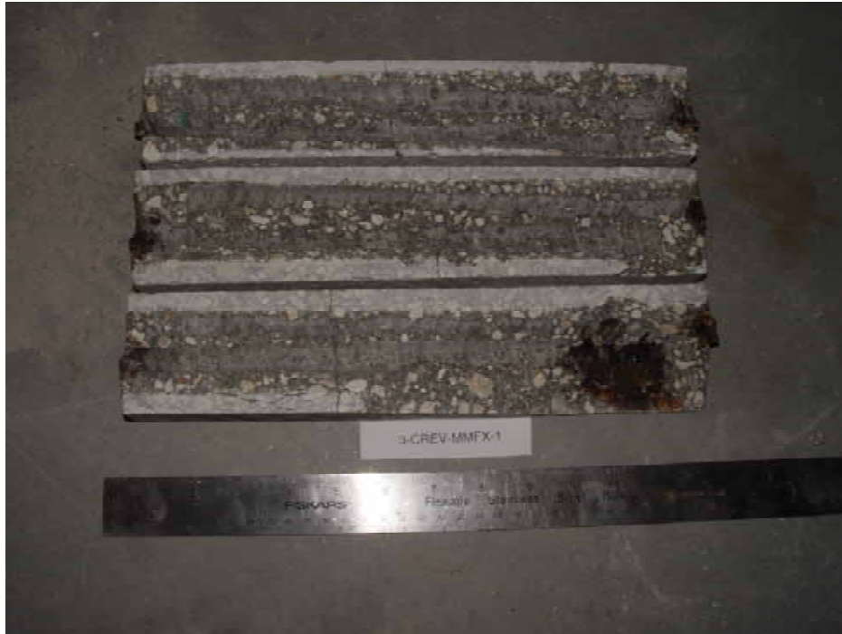
Figure 4.61. Photo. Trace of the upper rebar and corrosion products on specimen number 3-CREV-MMFX-1.
