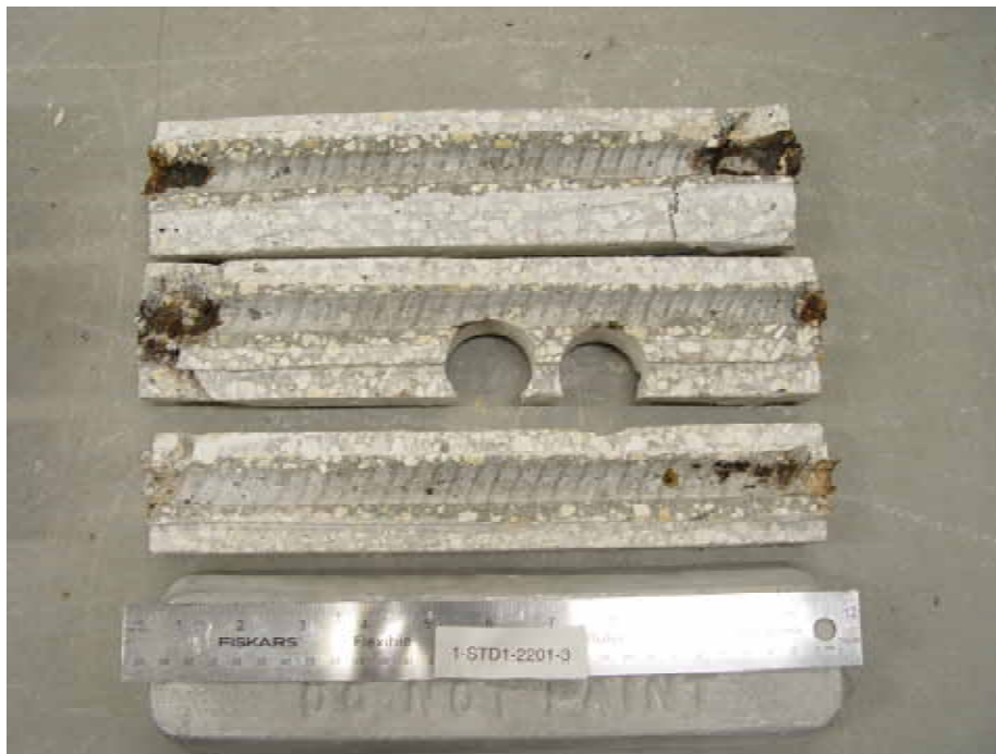
Figure 4.105. Photo. Trace of the upper rebar and corrosion products on specimen number 1-STD1-2201-3.
