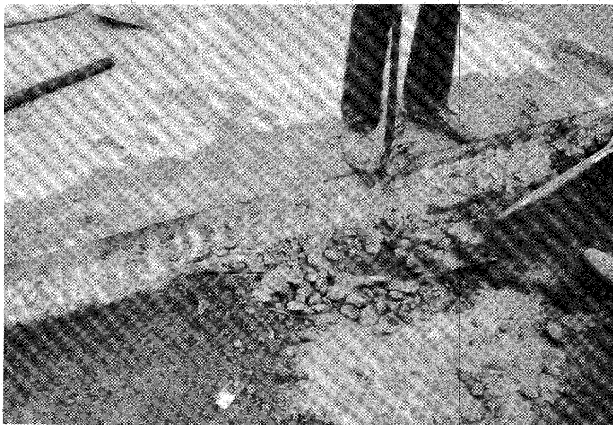
FIGURE 12 – CLEANING REPAIR AREA
