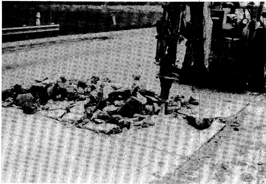
FIGURE 7 – BREAK CONCRETE Breaking concrete with pavement breaker.
