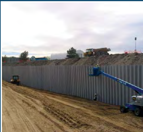
Installation of barrier wall
