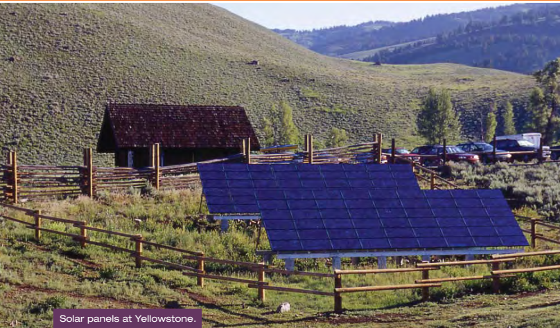
Solar panels at Yellowstone.
