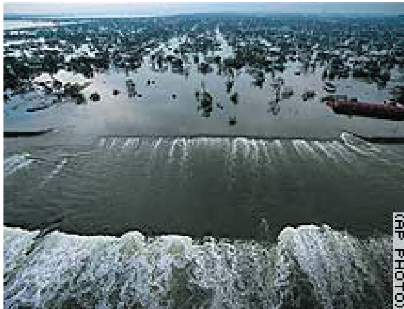
Figure 10. Levee breach allowing water from Lake Pontchartrain to pour into New Orleans.
