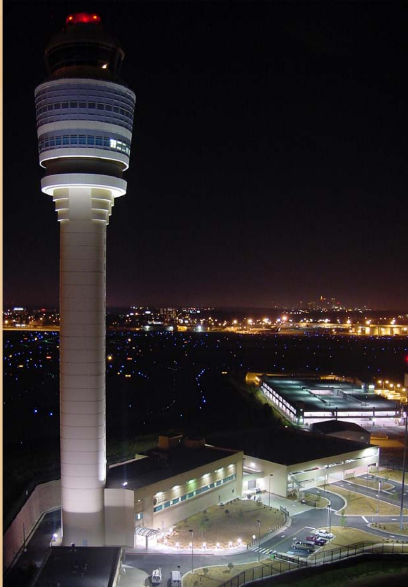
State-of-the-art air traffic control towers, like this one at Hartsfield-Jackson Atlanta International Airport, are helping air traffic controllers better guide current air traffic as well as accommodate future growth, making the safest aviation system even safer. Credit: Greg Haire, Airway Transportation System Specialist, Technical Operations, Hartsfield-Jackson Atlanta International Airport
