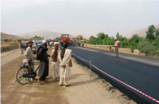
The paving of the Kabul Kandahar road in Afghanistan.
