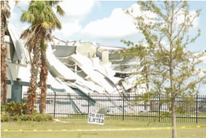
Florida building damaged by Hurricane Charlie.
