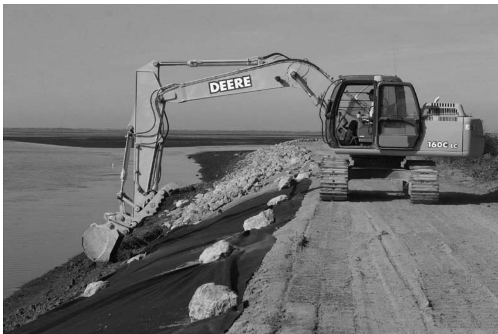
Erosion control and dike maintenance at Salmon Creek Unit.
