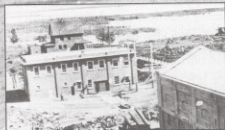
The old Minidoka Power House in 1909.
