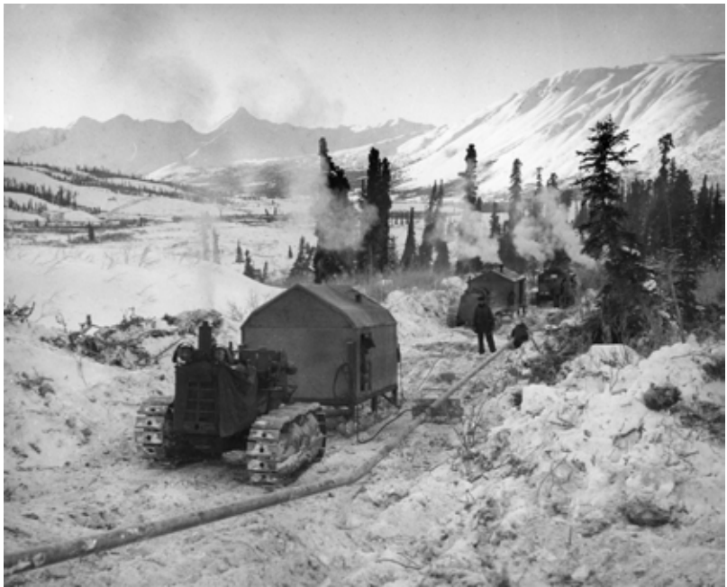
Pipeline welding the CANOL on Macmillian Pass.
