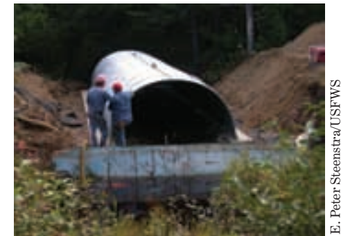
New culvert construction underway.
