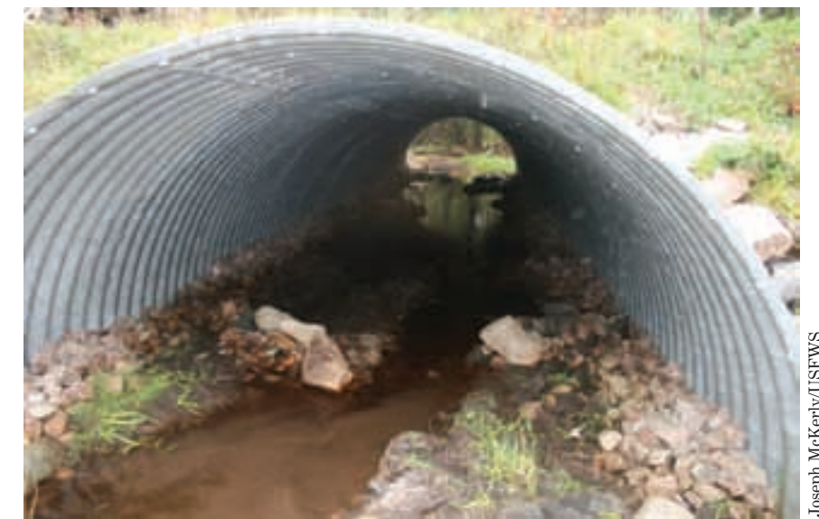
Fish habitat fills this arched culvert throughout its length, allowing Atlantic salmon, brook trout, turtles and aquatic bugs to pass under the road without hinderance.
