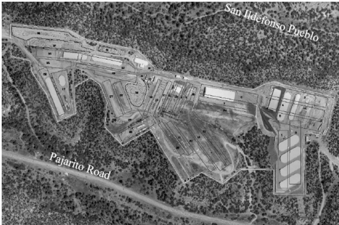
Figure I–15 Waste Management Areas within the Existing Area G Footprint in Technical Area 54
