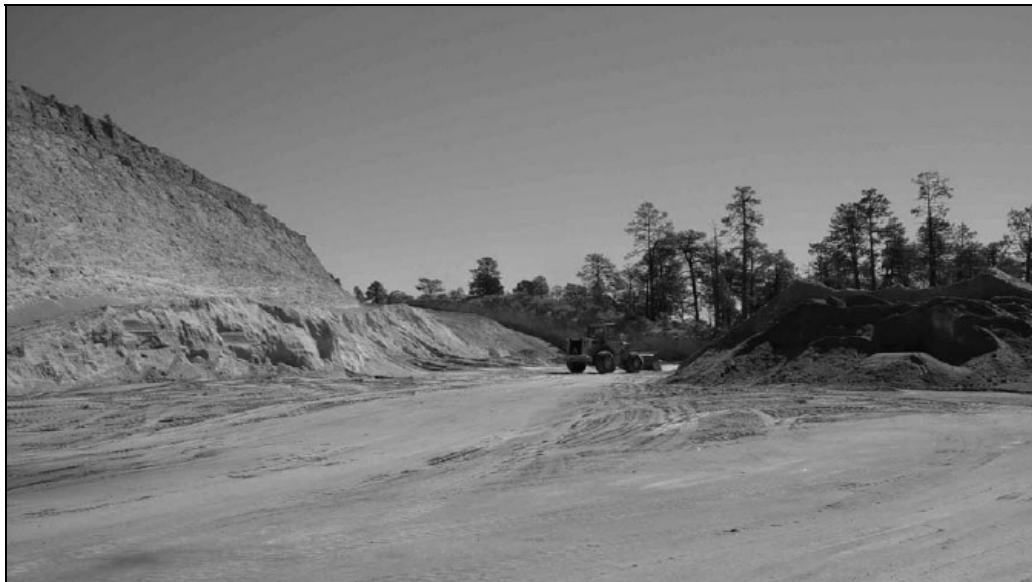
Figure I-23 View to the East from within the Technical Area 61 Borrow Pit
