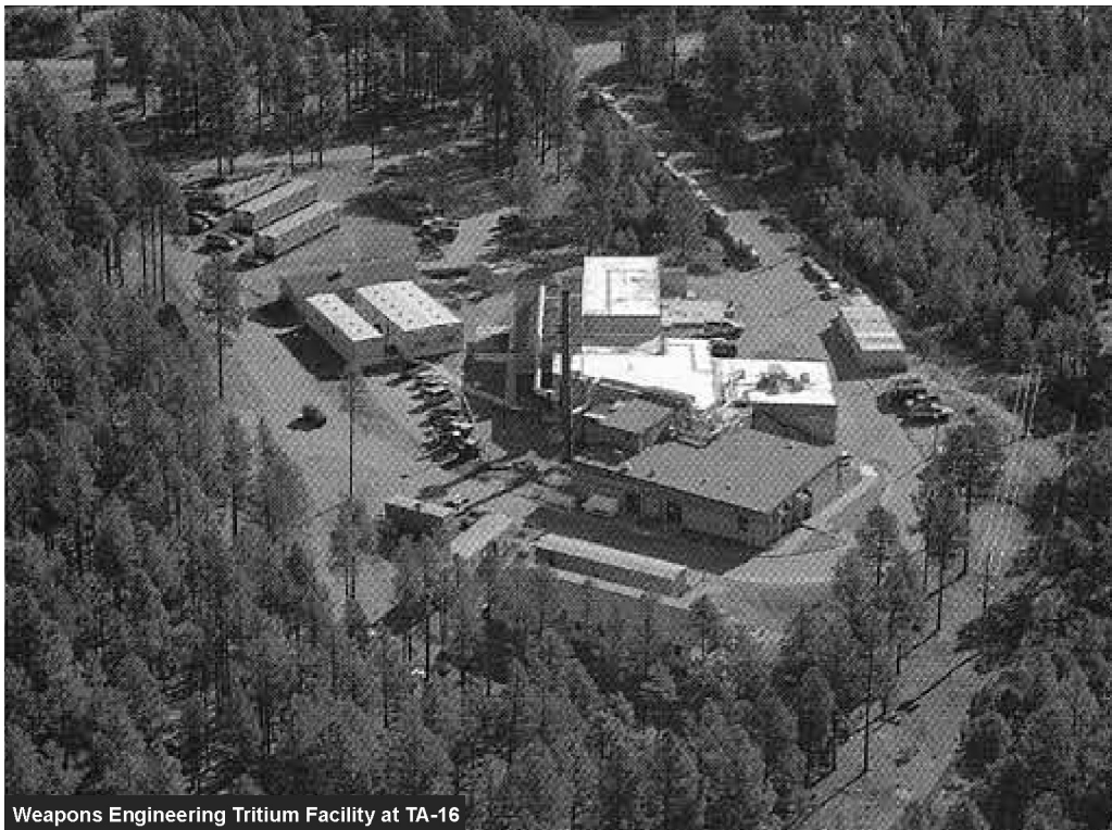
Weapons Engineering Tritium Facility at TA-16
