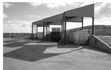
Transfer Station Built in Part with Grant Funds
