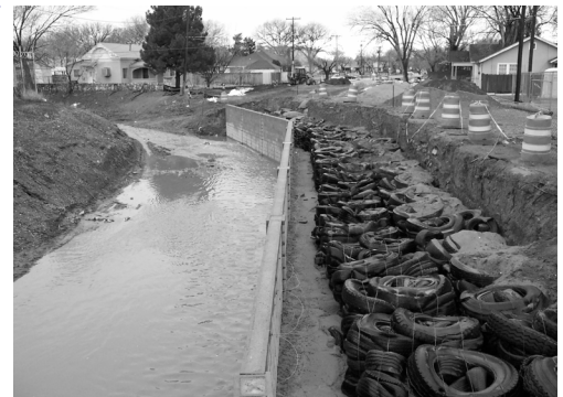
Baled tires used for erosion control
