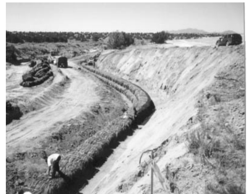
Baled tires used for bank stabilization at a closed landfill
