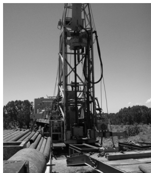
Installation of Groundwater monitoring wells is fundable
