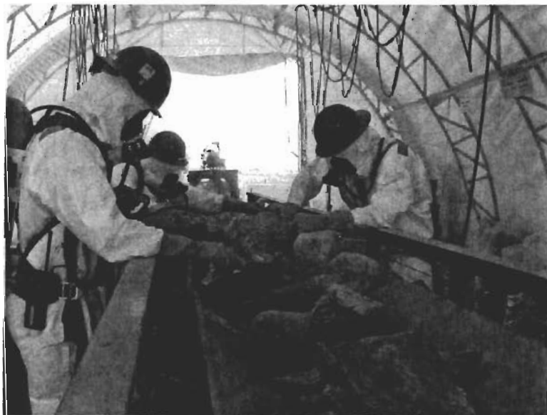
Figure 3-7 Debris Sorting on the Conveyor Belt in the Waste Management Tent Using Airline Respirators
