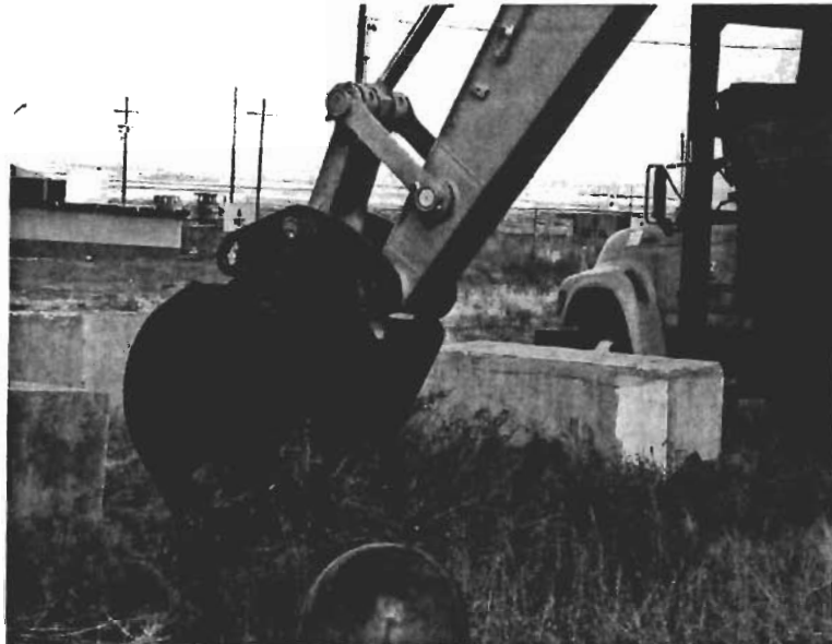
Figure 3-3 Trackhoe Begins Excavation
