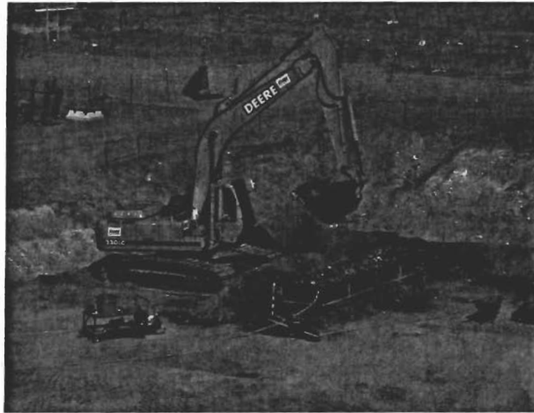
Figure 3-5 Trackhoe in Operation Using a Table Screen
