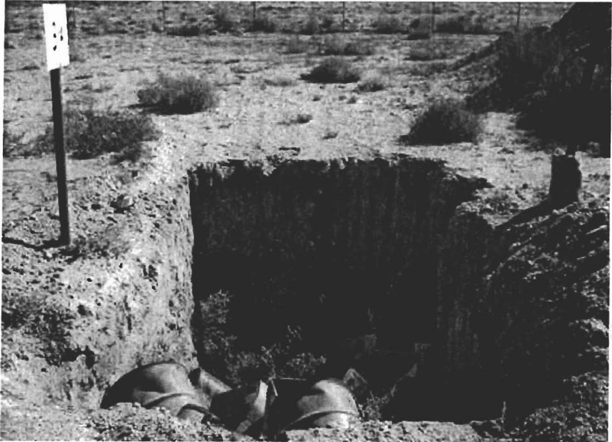
Figure 2-5 Historic Photograph Showing a Disposal Pit and Associated Marker
