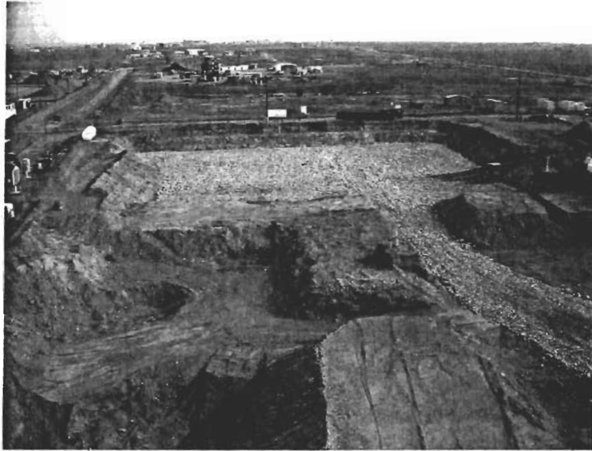
Figure 4-16 View of the Excavation Looking North with the Rock Layer in Place
