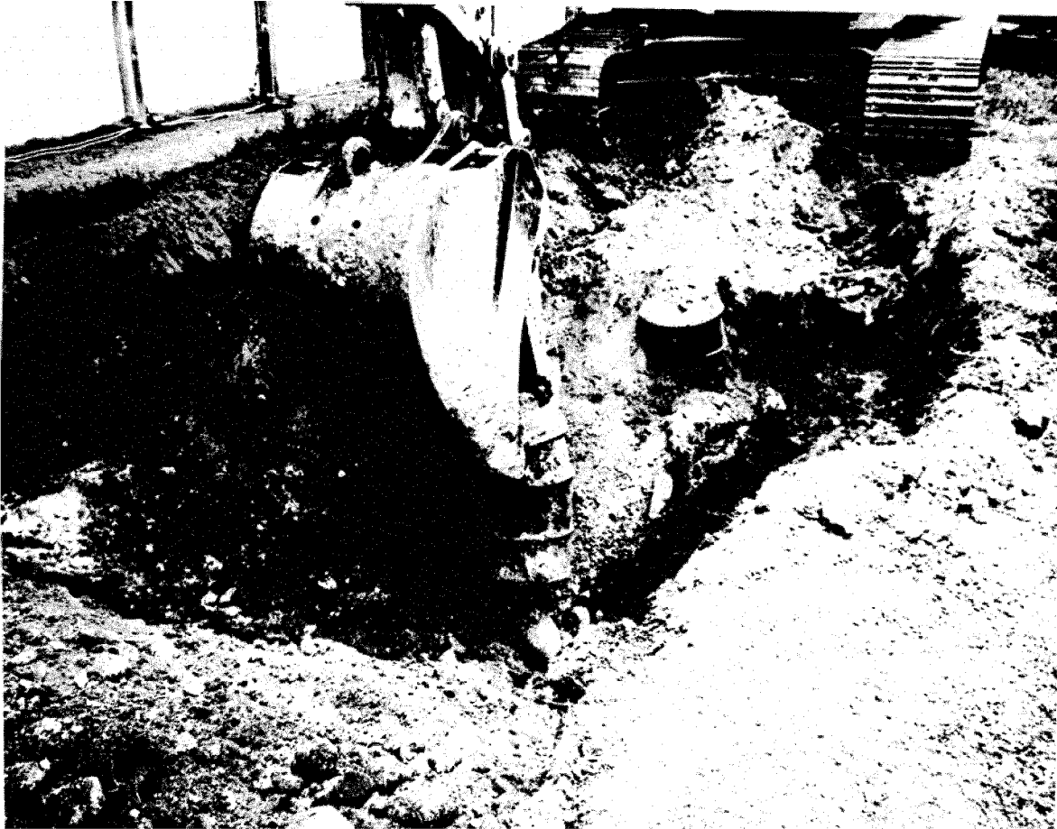
Figure A-2. Rocky Flats excavation.
