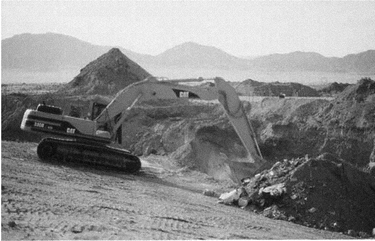
Figure A-1. Sandia Landfill excavation.
