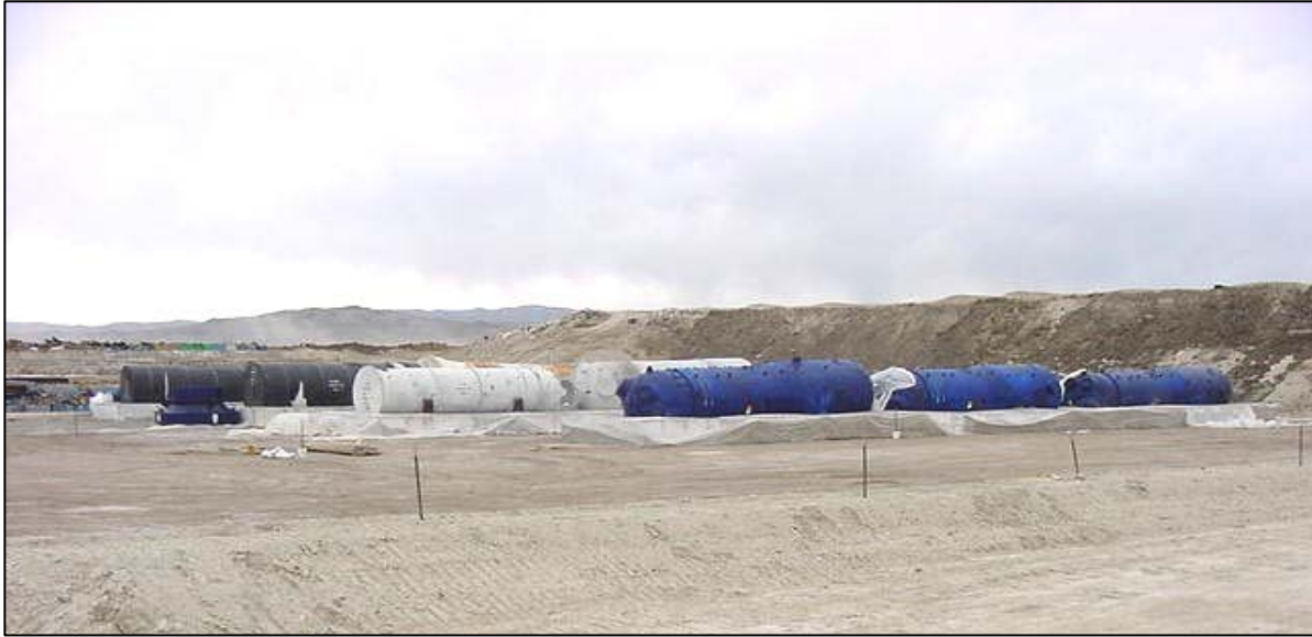
Figure 3-2. Large Component Disposal
