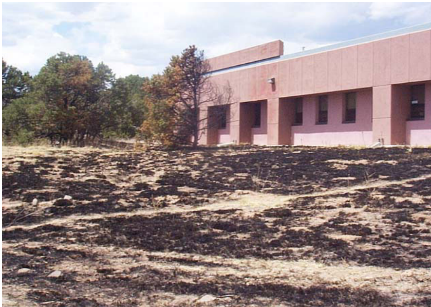
Figure 2-10. TA-46 Building 2 After the Cerro Grande Fire, 2000.
