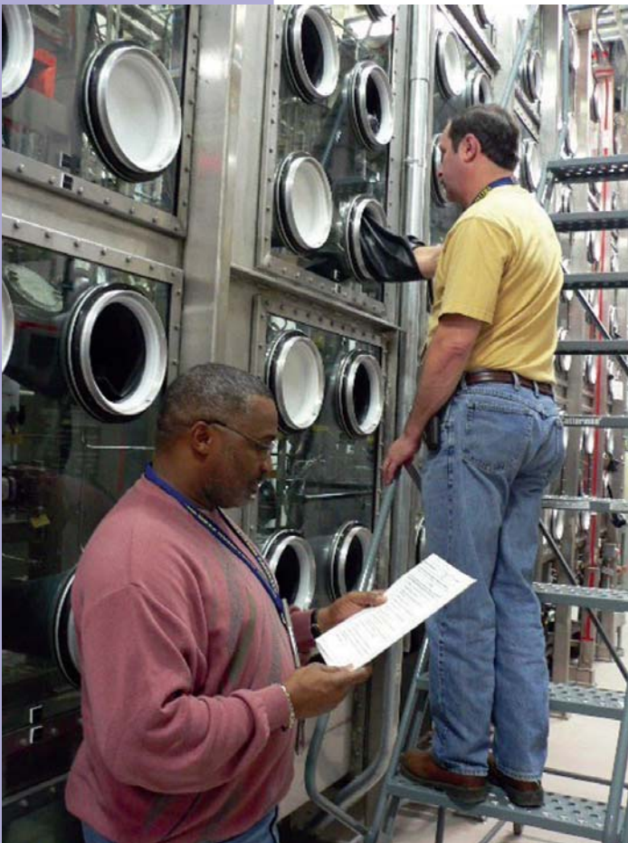
Examining material at the Tritium Extraction Facility.
