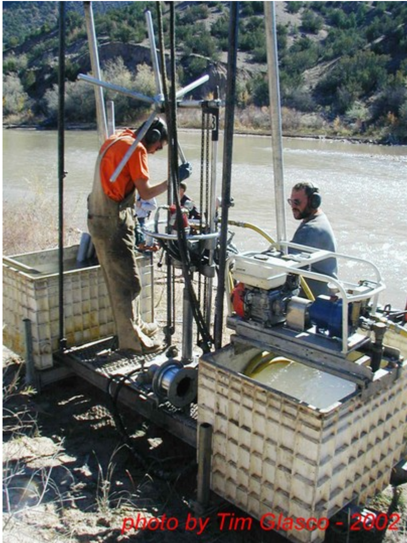
Test Drilling in White Rock Canyon - Fall 2002
