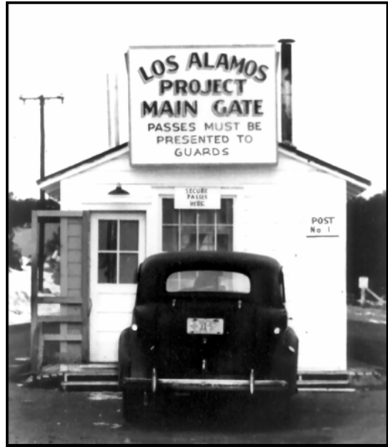
Figure1-4: An early photo of the main gate into Los Alamos
