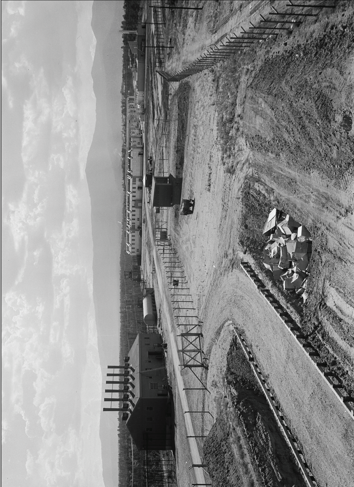
Figure 2.0-2. Waste disposal practices at MDA A circa late 1945; similar trench conditions and waste disposals are assumed to have existed at MDA B during this time period (LANL photograph IM-9: 2284)
