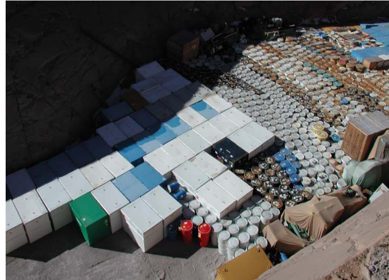
Low-level waste disposal in Pit 38
