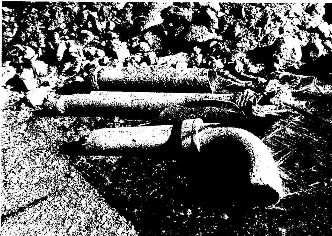
Photo I-6: Sections of outfall pipe.
