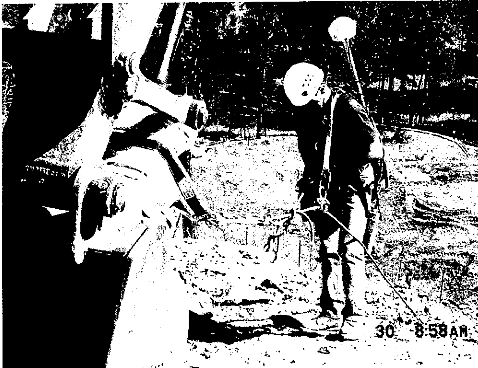
Photo I-27: Rigging fall protection to excavator before starting slope survey.
