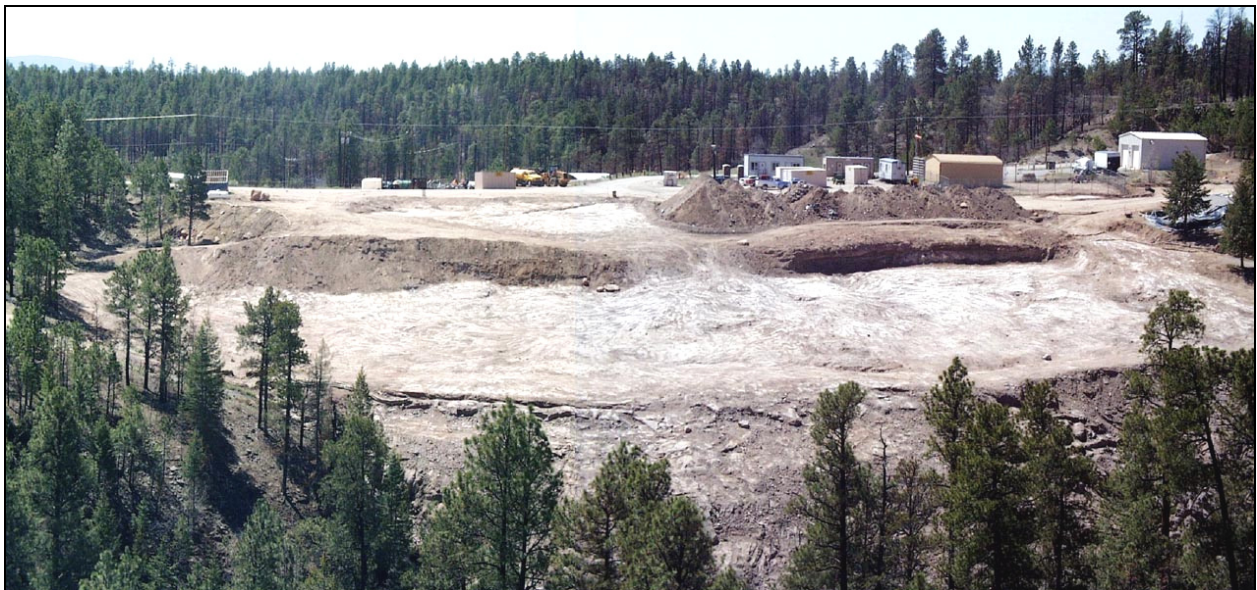
Photograph 1.4-2. Post-excitation condition of the MDA P Site
