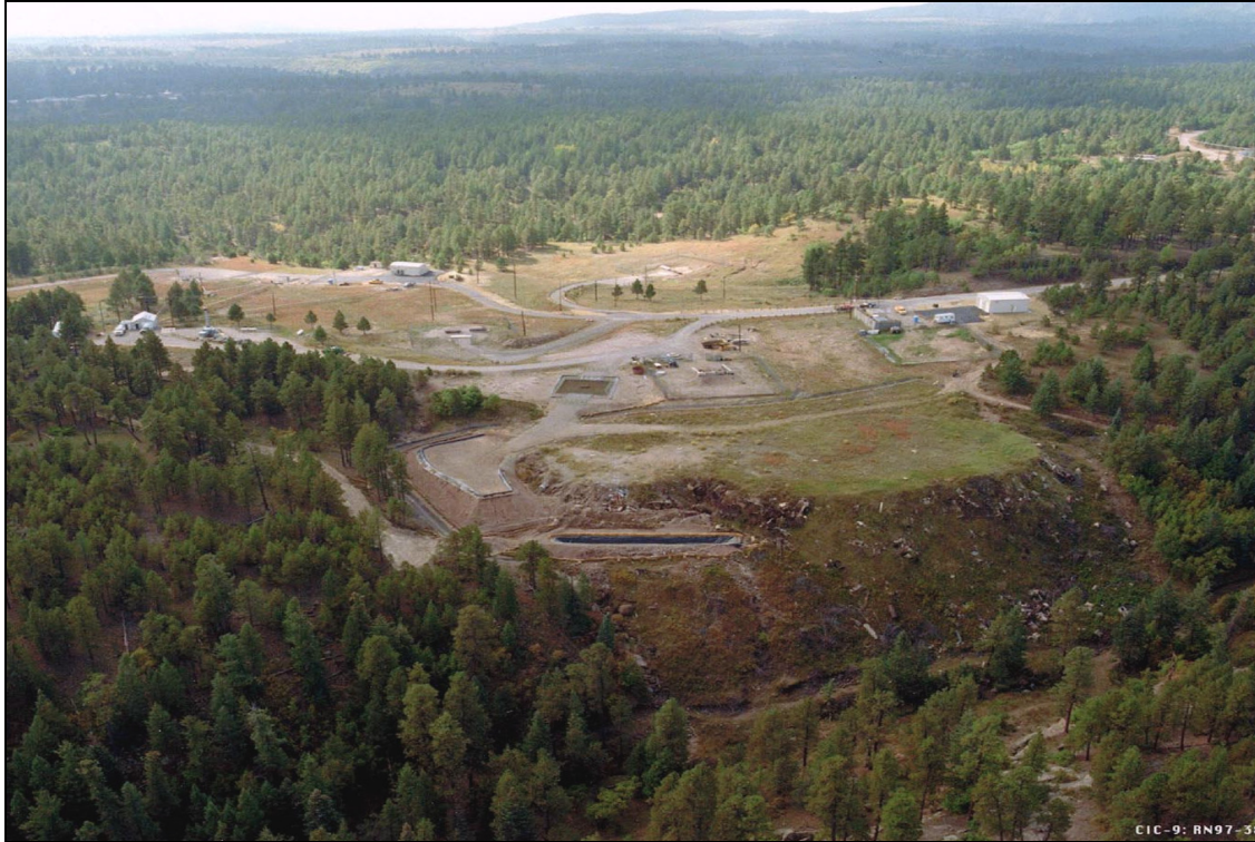
Photograph 1.4-1. Aerial view of the MDA P Site prior to excavation, 1997
