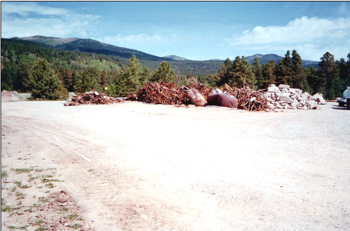
Photograph 2.2-6. Example of metal and concrete debris, post-segregation, 1999
