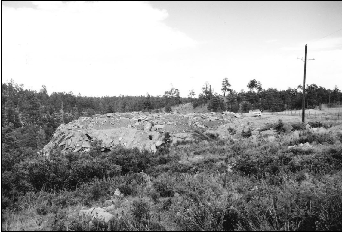
Photograph 1.4-5. West lobe of MDA P (debris from 1960s burning as well as concrete from 1970s deconstruction of Building 260), 1973
