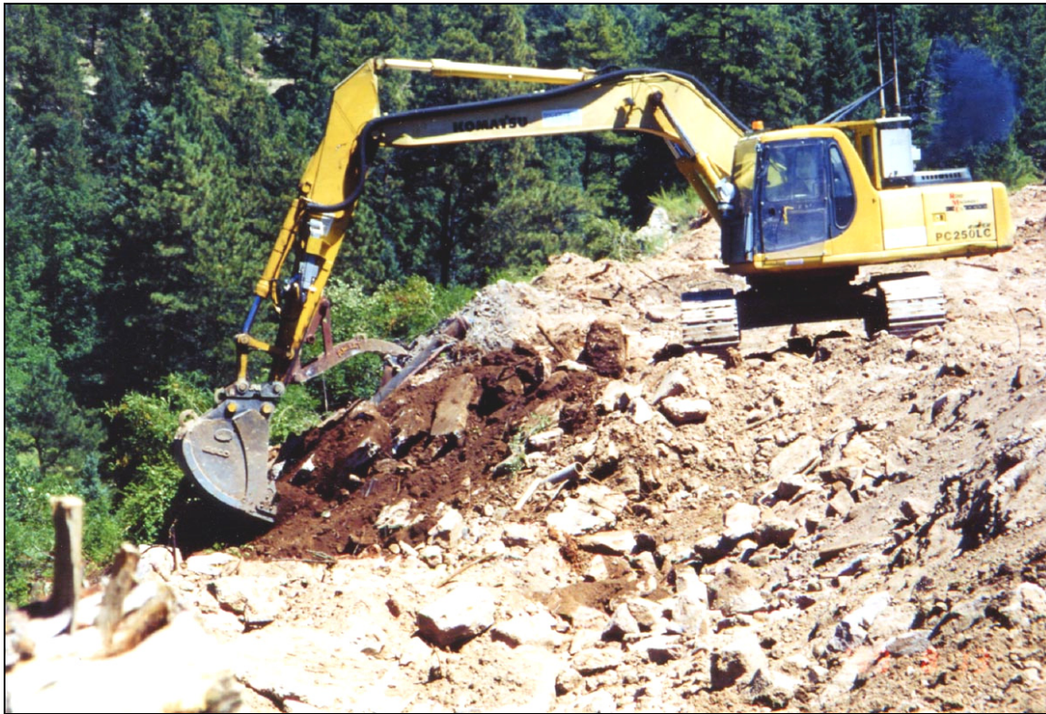
Photograph 2.2-1. Remote excavation of MDA P contents, 1999 (view to east)
