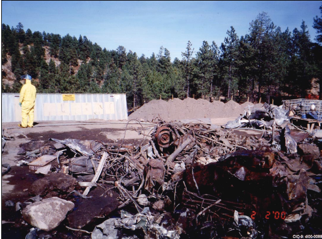
Photograph 2.2-4. Example of excavated materials, shown during segregation process, 2000 (view to northeast)
