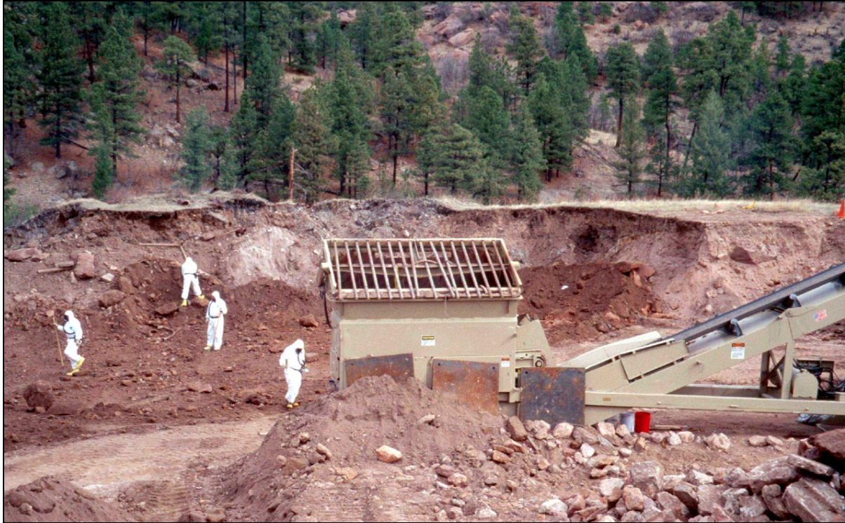
Photograph 2.2-5. Soil excavation (over-excavation)
