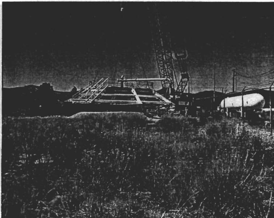
Photograph 2. Crane lowering off-gas hood, MDA V
