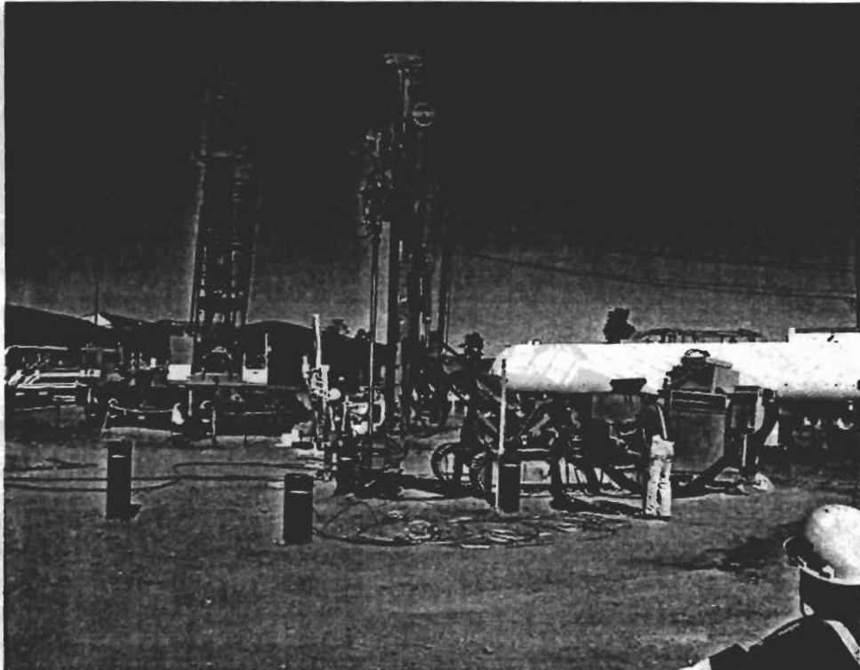
Photograph 1. Installation of electrodes at the hot demonstration site, MDA V
