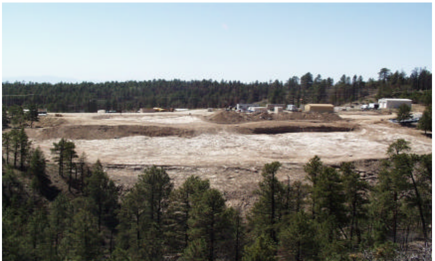
Material Disposal Area P after cleanup activities
